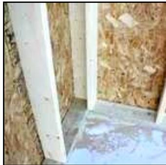
Instead, use a two-stud detail with non-structural backing to support the drywall as allowed per CBC 2308.9.2. Backing can be wood, specified sheathing or panel materials, and “other approved devices”.
