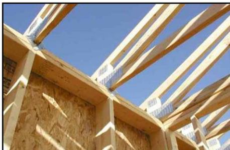
*Raised heel roof trusses*
